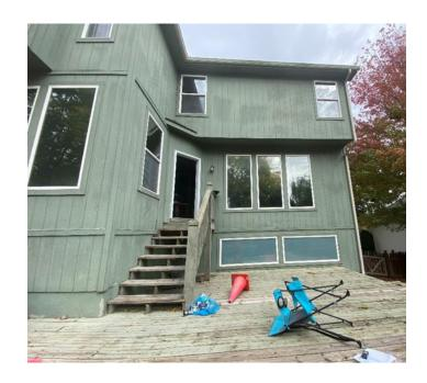
Scope of Work- Remove 17'  $\times$  25' Wood Deck on back of house. Build a 12'  $\times$  15' Covered Screened in Deck that walks out at the same height as the current Back Door. Install Electrical Lights, Switch and Outlets.
