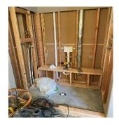
Scope of Work- Remodel Master Bathroom to include Install New: Walk-In Shower with New Concrete Base, Tile Walls and Floor, Niche, Accent Stripe, Light, Quartz Bench with Tile Facing. Center both the LED Ceiling Light over the Shower & center both Shower Faucets. Install New: Tile Flooring; Tile Backsplash behind Vanity & Jacuzzi; Tile around Jacuzzi. Finish Ceiling with Smooth Finish. Install 2 new Lights over the current Vanity. Set new Stool. Remove 2 Sink Faucets & Jacuzzi Faucet.
